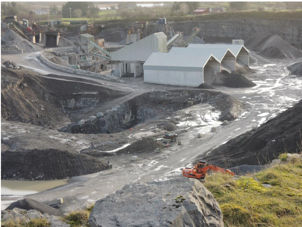
Figure 8: Preparation for further blasting in south quarry 19 th December 2015
