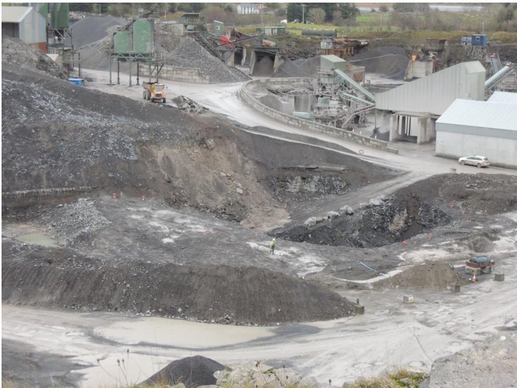
Figure 6: Preparation for further blasting in south quarry 18 th December 2015
