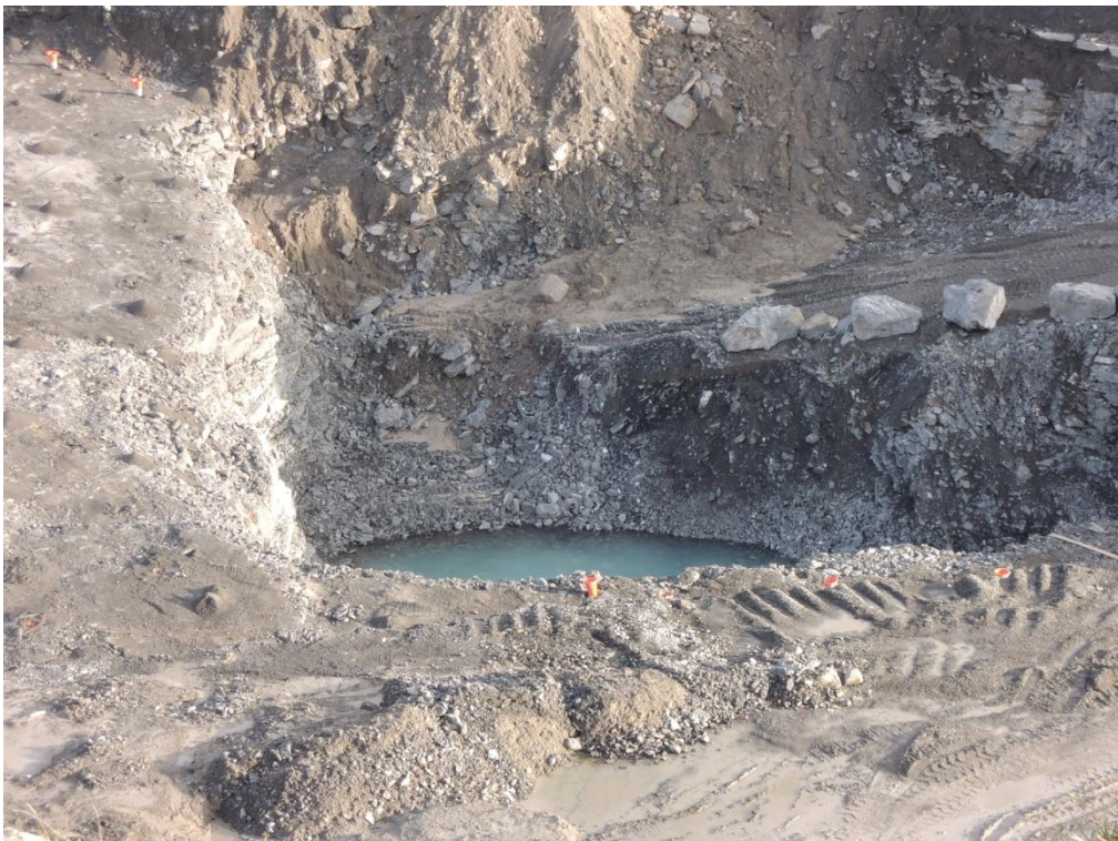
Figure 10: Preparation for further blasting in south quarry 19 th December 2015 - Blast took place in early January 2016
