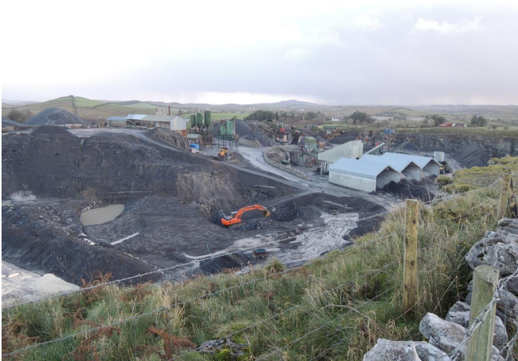
Figure 4: New excavation in south quarry of quarry floor progressing 29 th November 2015
