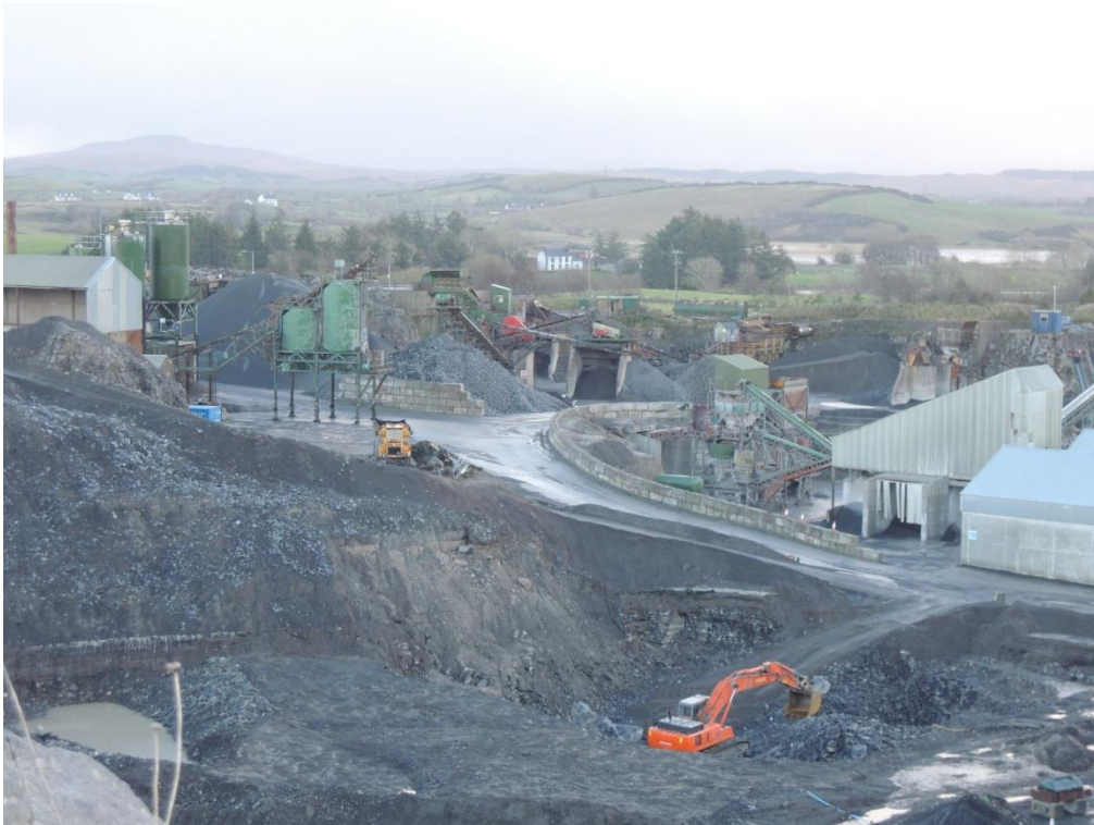
Figure 5: New excavation in south quarry of quarry floor progressing 29 th November 2015
