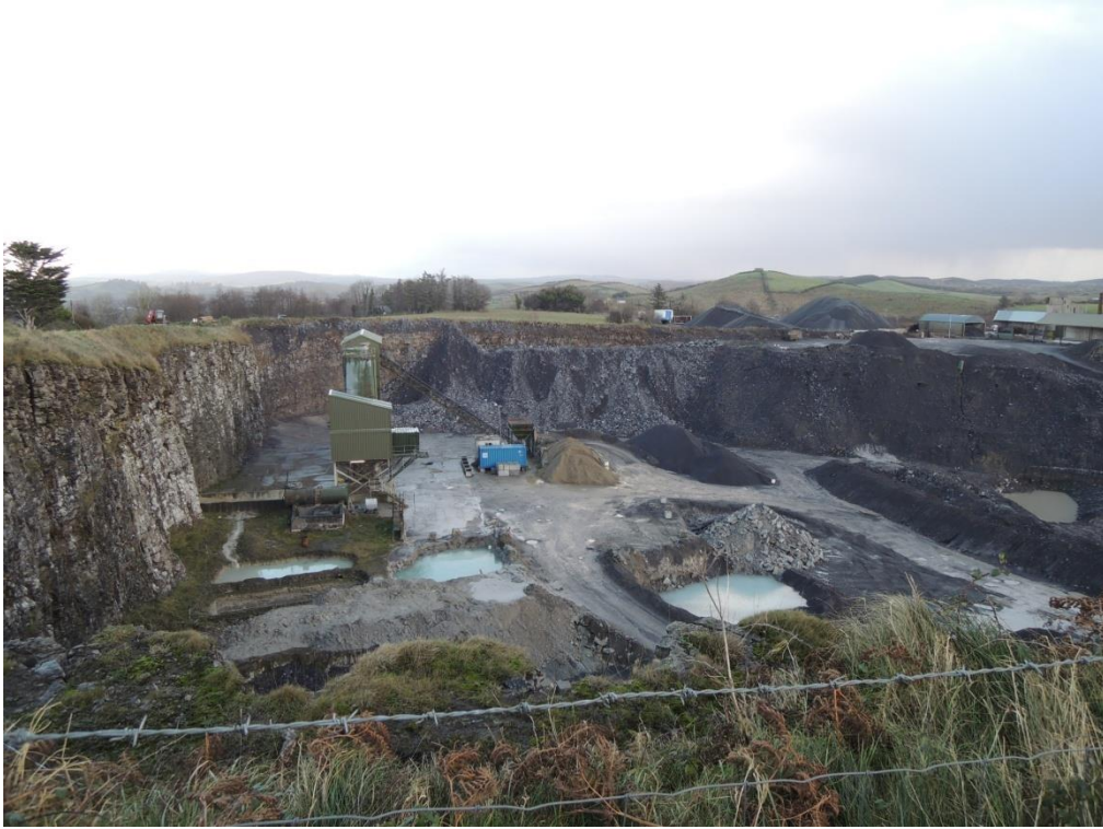
Figure 3: New excavation pits in south quarry 29 th November 2015
