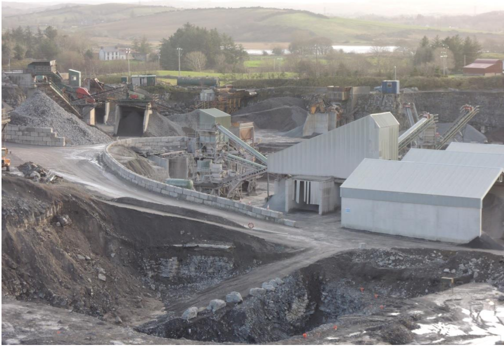
Figure 9: Preparation for further blasting in south quarry 19 th December 2015
