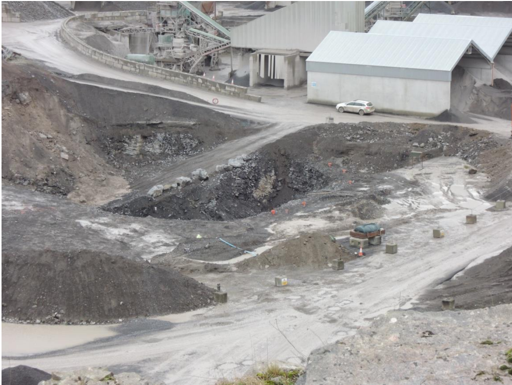
Figure 7: Preparation for further blasting in south quarry 18 th December 2015
