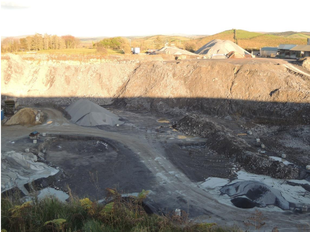
Figure 2: south quarry - new excavation of quarry floor in centre right of photograph 31 st October 2015
